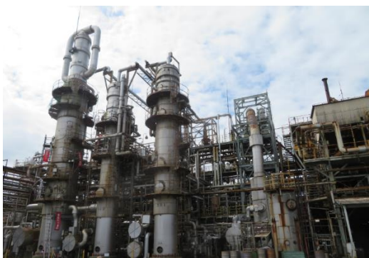
The TDI plant in Omuta Works
