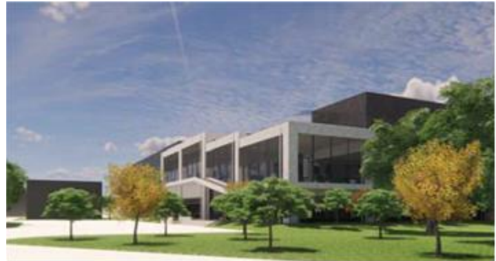
Illustration of facility exterior
